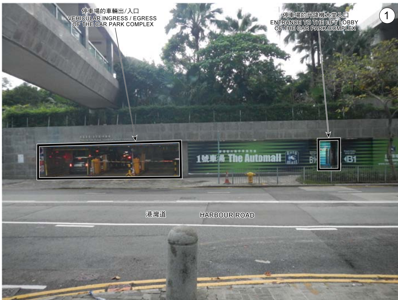
面向港灣道的車輛出/入口及大堂入口 VEHICULAR INGRESS / EGRESS AND ENTRANCE FACING HARBOUR ROAD
