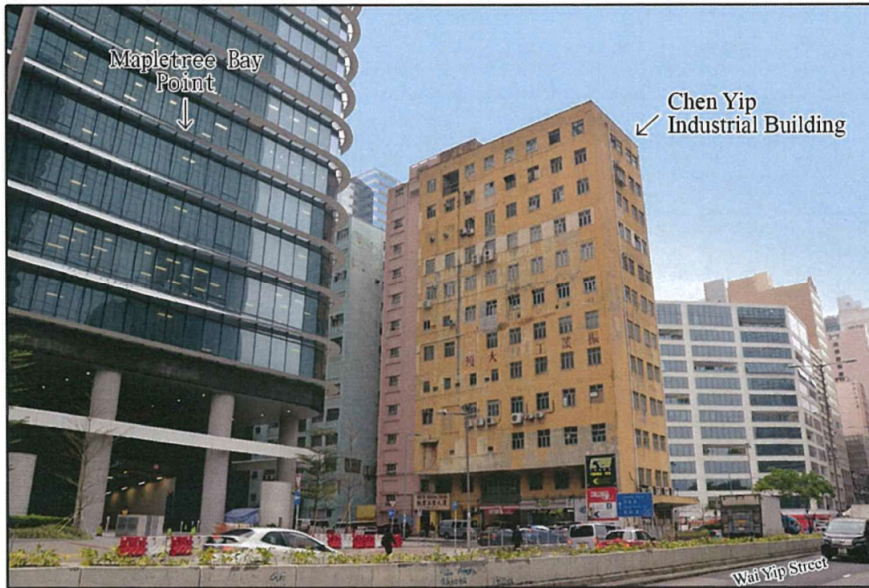
Photo 3A Existing Condition at the Subject Site
