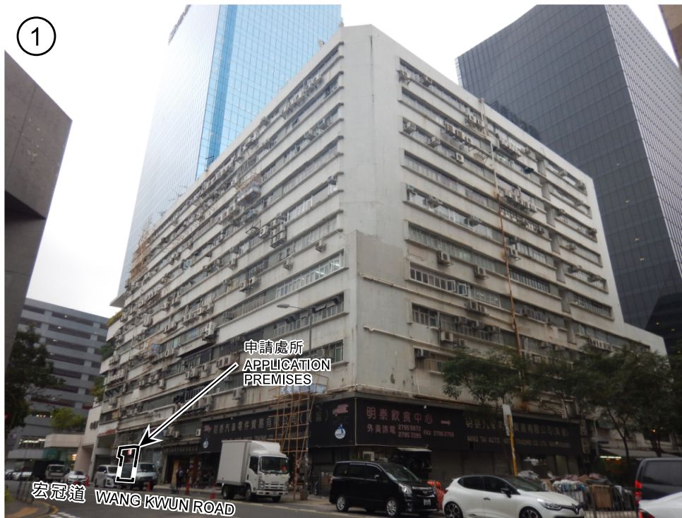
有關樓宇 THE SUBJECT BUILDING
