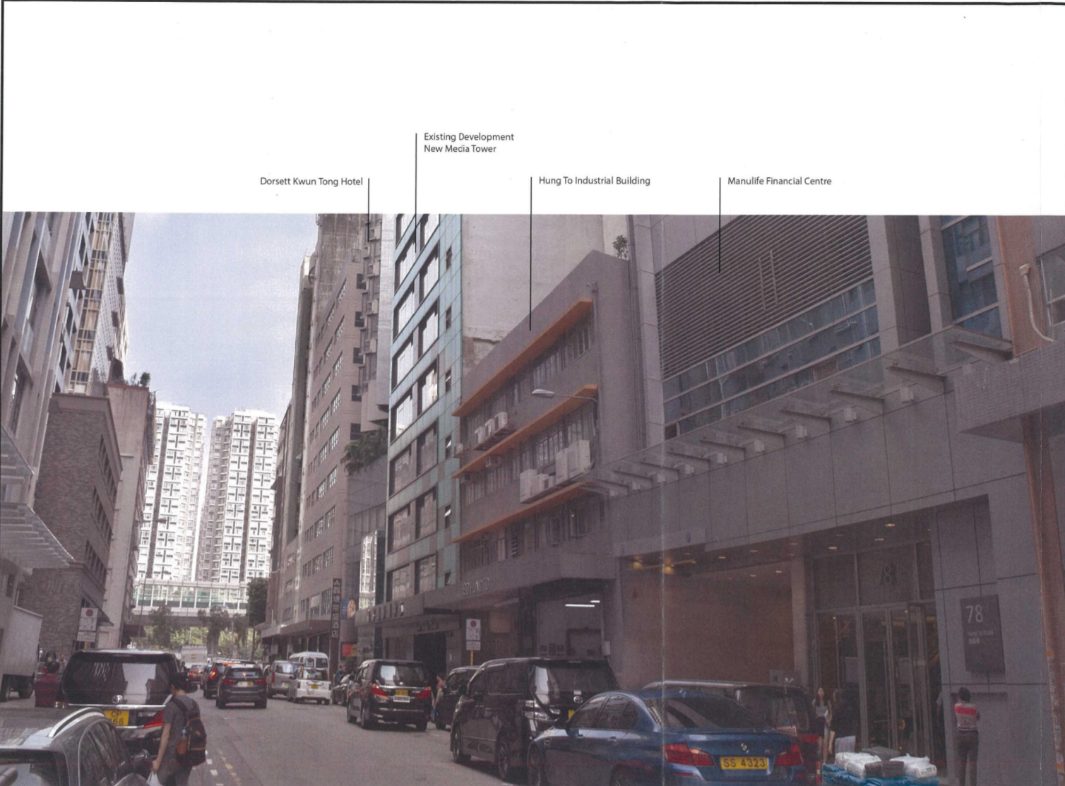
VP 02: View south east along Hung To Road towards the Application Site (existing situation)
