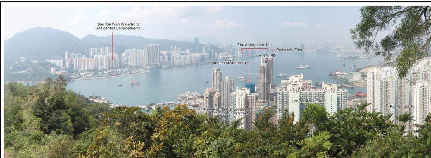
Existing View (March 2019)
