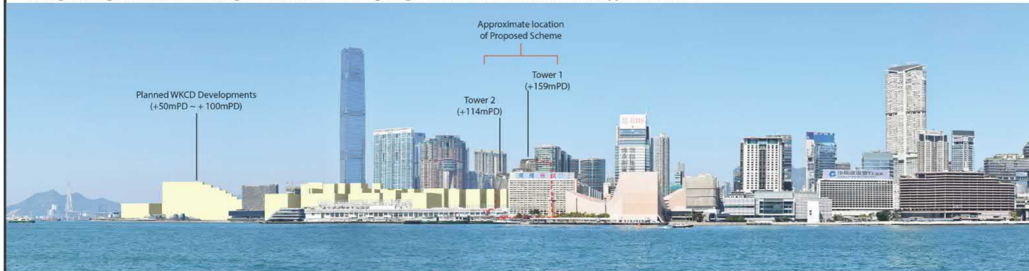
Strategic Vantage Point 03: View looking north-west from the Hong Kong Convention and Exhibition Centre (Year 10)
