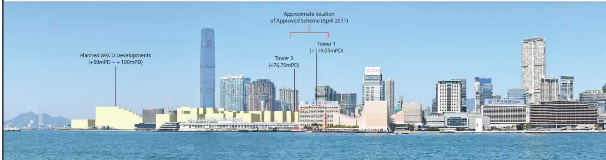
Strategic Vantage Point 03: View looking north-west from the Hong Kong Convention and Exhibition Centre (Approved Scheme)
