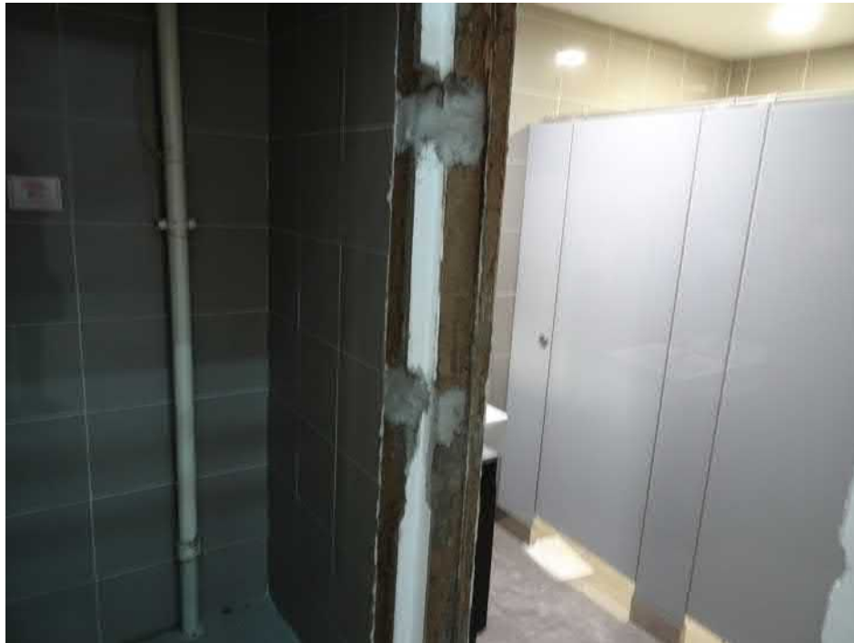
申請處所內部 INTERIOR OF APPLICATION PREMISES
