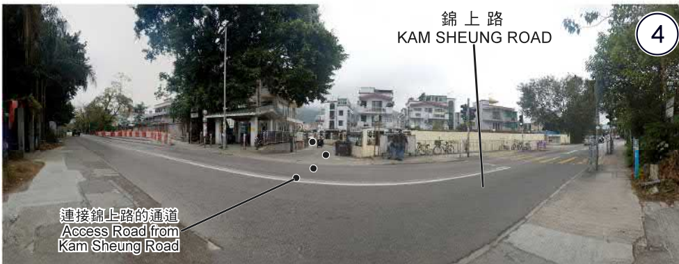
連接錦上路的通道 Access Road from Kam Sheung Road
