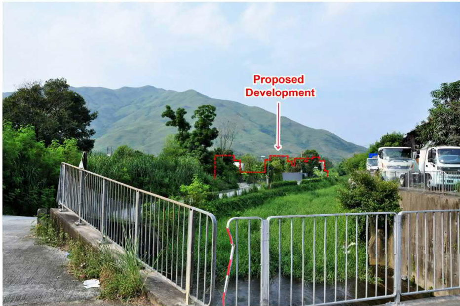
Photo 2 Proposed Development at the Application Site
