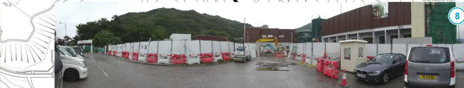
有機資源回收中心 (第一期) (興建中) ORGANIC RESOURCES RECOVERY CENTRE (PHASE I) (UNDER CONSTRUCTION)
