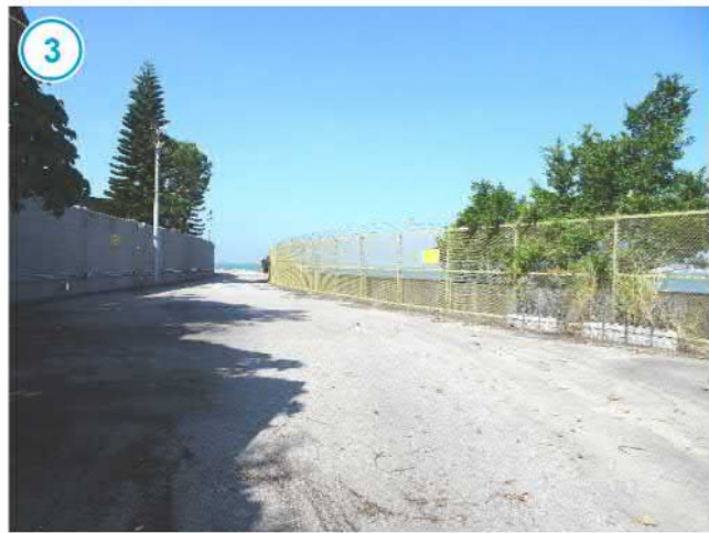
深水角氯氣裝卸區 SHAM SHUI KOK CHLORINE LOADING AND UNLOADING AREA
