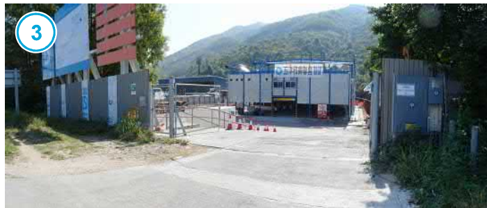
渠務署的臨時工地 TEMPORARY DRAINAGE SERVICES DEPARTMENT WORKS AREA
