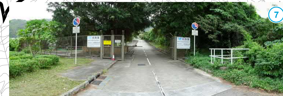
小蠔灣濾水廠入口 ENTRANCE OF SIU HO WAN WATER TREATMENT WORKS
