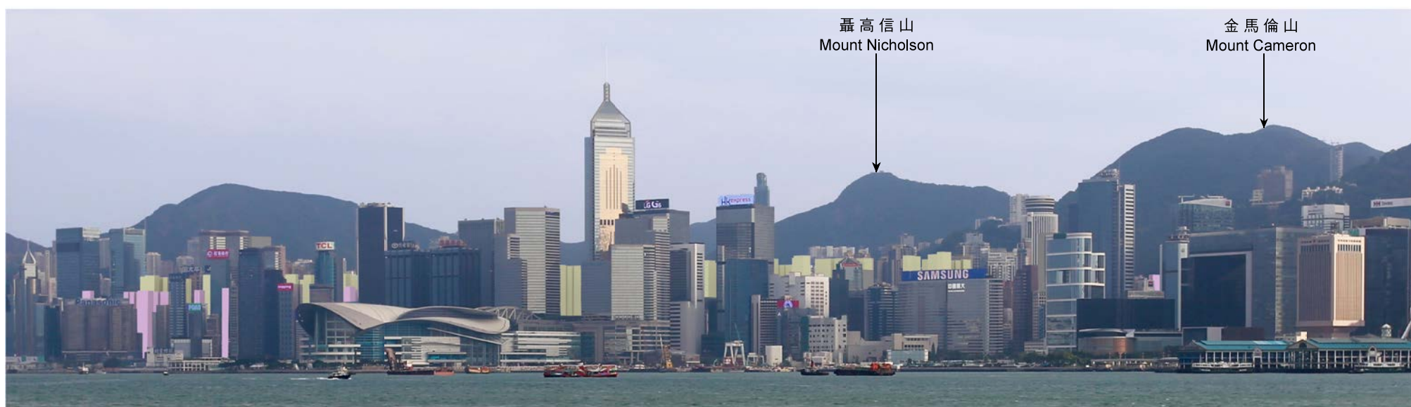
擬議的建築物高度限制 PROPOSED BUILDING HEIGHT RESTRICTIONS 110mPD 135mPD 已批准之發展 COMMITTED DEVELOPMENT
