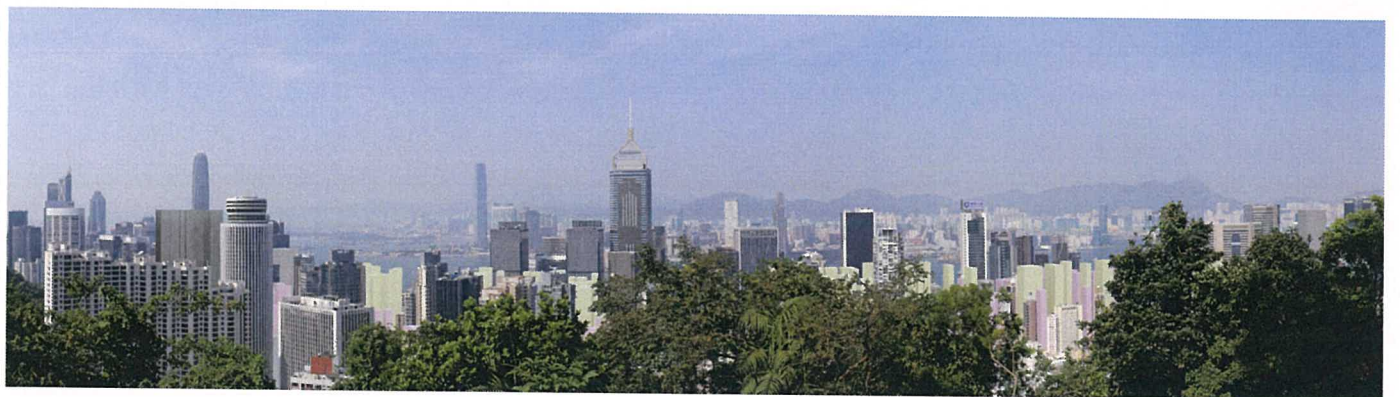
擬議的建築物高度限制 PROPOSED BUILDING HEIGHT RESTRICTIONS 110mPD 135mPD 已批准之發展 COMMITTED DEVELOPMENT
