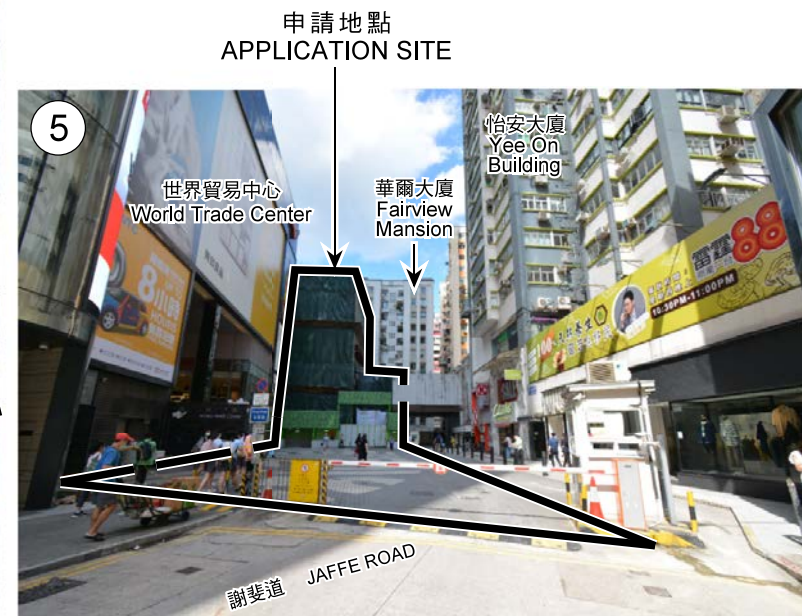
從謝斐道東方向望向申請地點的景觀 EASTERN VIEW OF THE APPLICATION SITE FROM JAFFE ROAD
