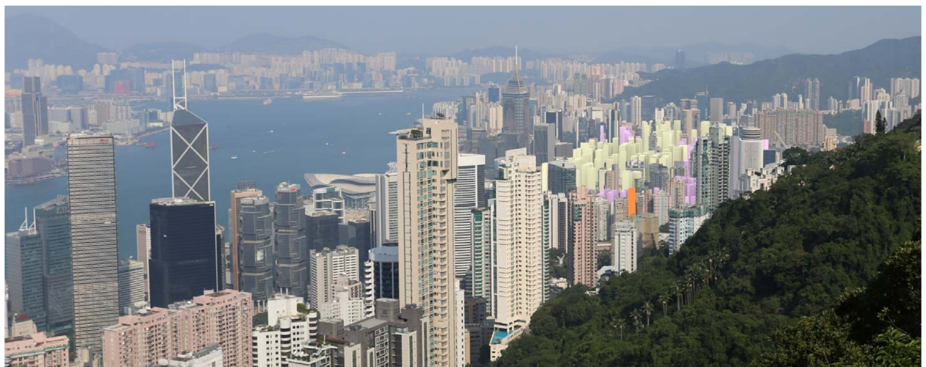
現時在灣仔分區計劃大綱草圖編號S/H5/28的建築物高度限制 CURRENT BUILDING HEIGHT RESTRICTIONS IN THE DRAFT WAN CHAI OZP No. S/H5/28
