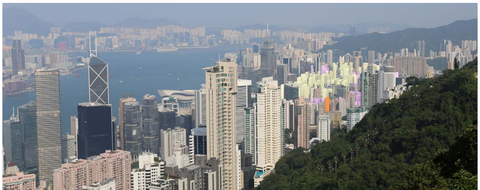
現時在灣仔分區計劃大綱草圖編號S/H5/28的建築物高度限制 CURRENT BUILDING HEIGHT RESTRICTIONS IN THE DRAFT WAN CHAI OZP No. S/H5/28
