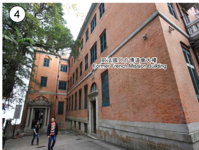
前法國外方傳道會大樓 Former French Mission Building
