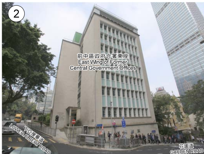
前中區政府合署東座 East Wing of Former Central Government Offices
