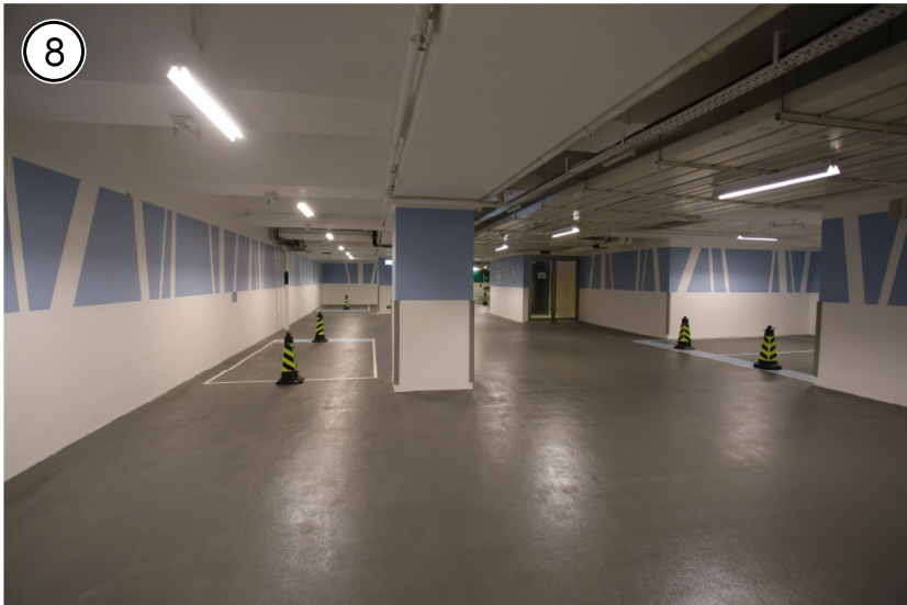
地庫一樓停車位及電梯大堂(可直達申請處所) CAR PARKING SPACES AND LIFT LOBBY (WITH DIRECT ACCESS TO THE APPLICATION PREMISES) ON BASEMENT 1/F
