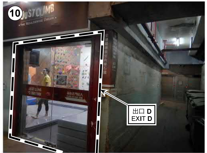
10 通往公用通道的出口 (擬議永久關閉) EXIT TO COMMON PASSAGE (PROPOSED TO BE CLOSED PERMANENTLY)
