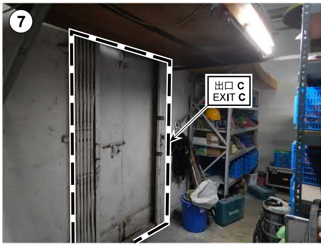
7 通往公用通道的出口 (擬議永久關閉) EXIT TO COMMON PASSAGE (PROPOSED TO BE CLOSED PERMANENTLY)
