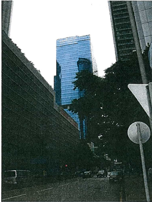
Figure 3i Views of Wang Tai Road (a key breezeway) Looking Northward (Image source: CO 2 nnsulting Ltd.)
