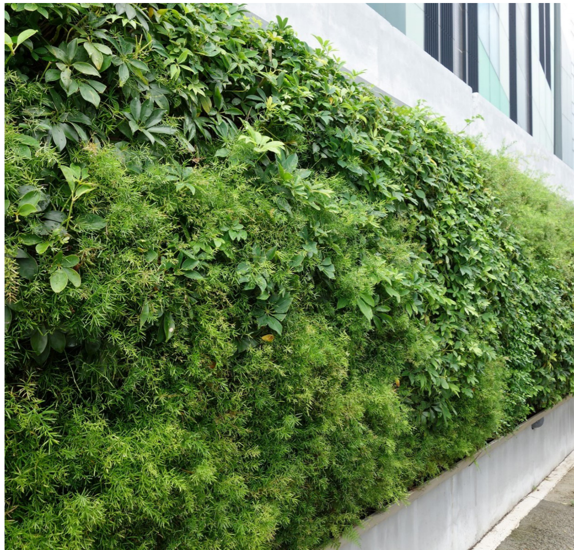
Fence wall for a project in Hing Kong utilising a similar tray system for the vertical greening.
