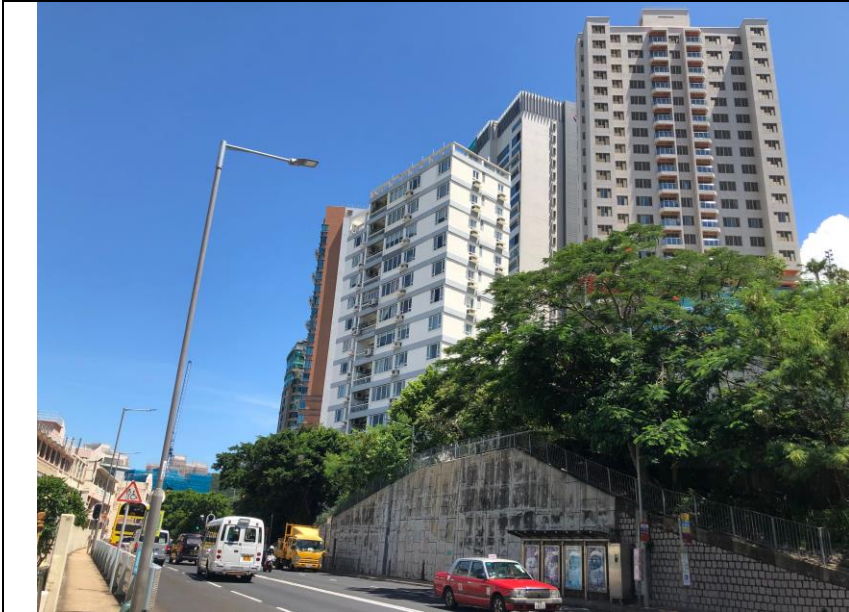
Figure 6: High rise, high-quality residential buildings opposite the application site on Pok Fu Lam Road
