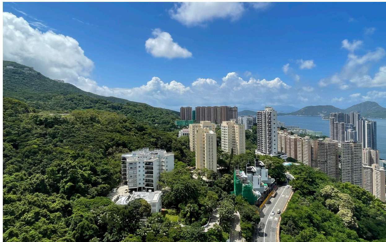
B View looking south east along the Pokfulam Road corridor showing the associated high-rise development
