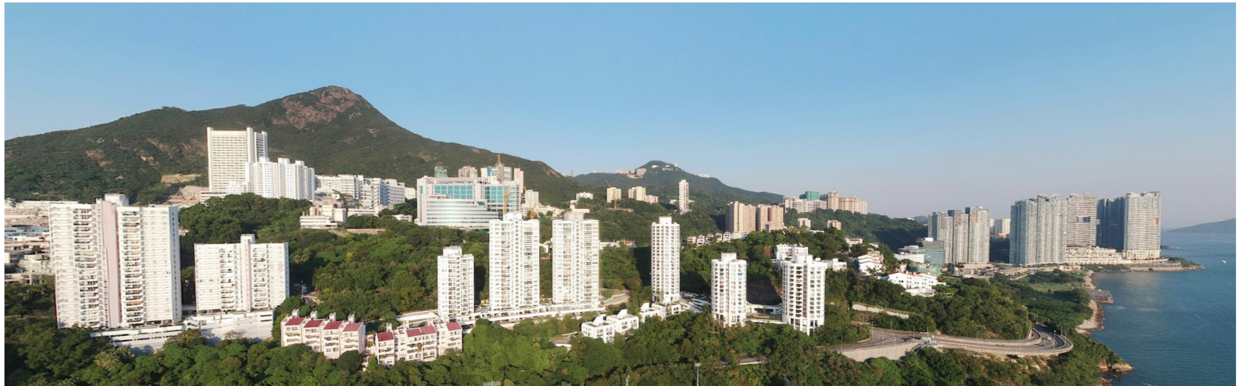
A View looking north east towards the Application Site demonstrates the scale of the landscape and visual setting and the importance of the mountain backdrop
