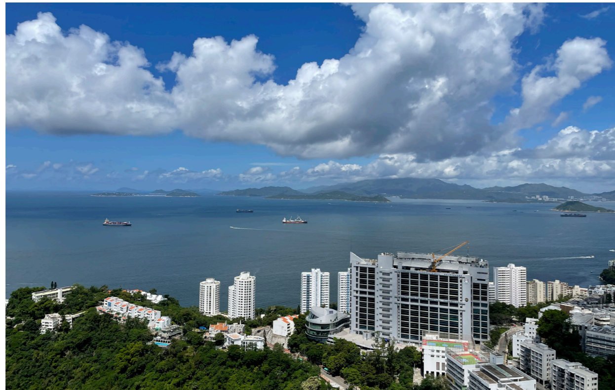
D E Key buildings controlling the visual envelope
