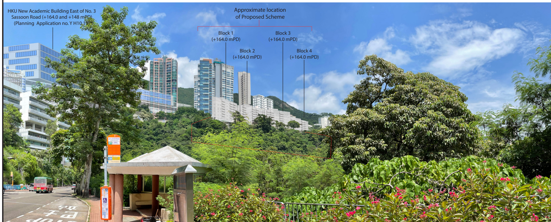
Vantage Point 05: View looking north east from Victoria Road (Year 10 with HKU New Academic Building at No. 3 Sassoon Road)
