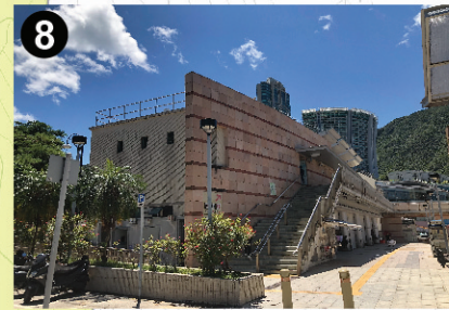
8 Repulse Bay Beach Building
