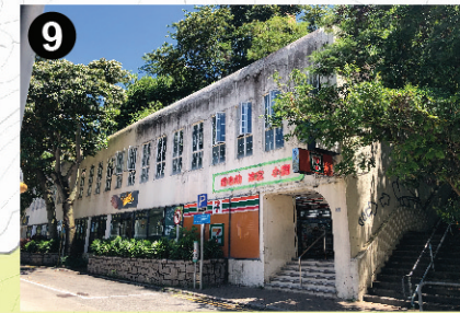
9 Beach Centre, a neighbourhood shopping centre on Beach Road
