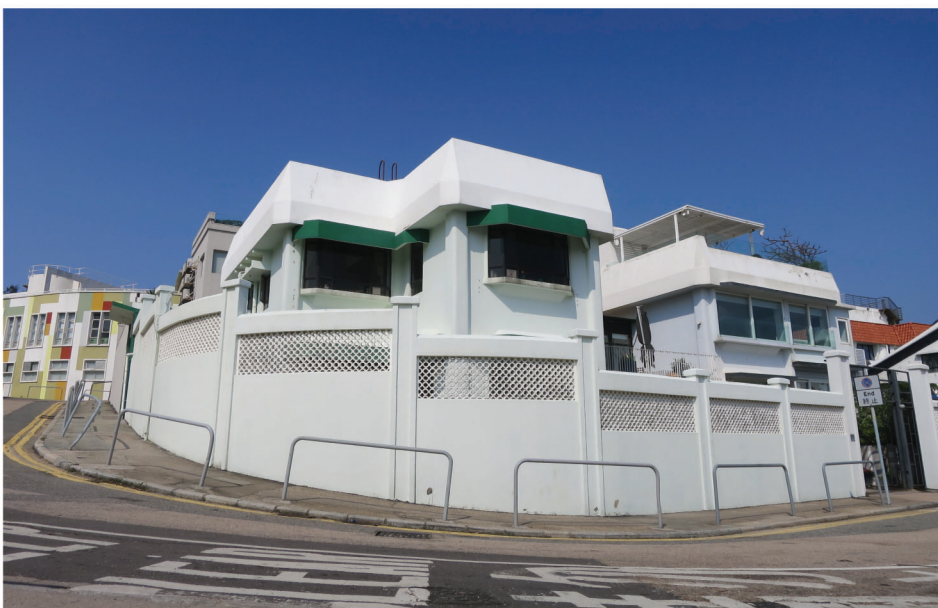
VP2 View from Hoi Fung Path Developments adjoining the Application Site on Stanley Link Road
