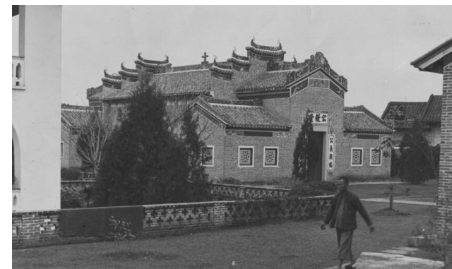
Fig 24: The Chapel at Loting (now Luoding), (Source: Fr. Kennelly, 'The chapel at Luoding, China, 1932', USC Maryknoll Mission Archives, UC1820088).
