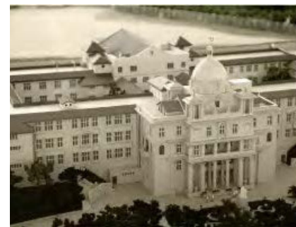
Fig 35: La Salle College, school inaugurated 1932, demolished 1970s
