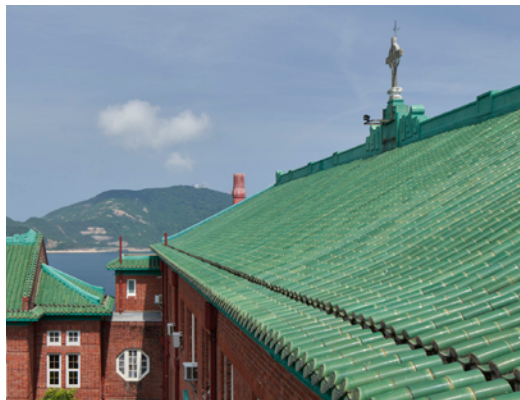
Current condition of existing building
