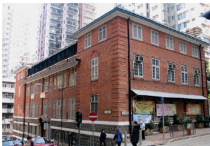
Fig 31: Main Building Old Tsan Yuk Maternity Hospital, completed 1922, Grade 1 (2009), (Source: AMO, 'Historic Buildings' [website], accessed 12 August 2024).
