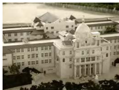
Fig 35: La Salle College, school inaugurated 1932, demolished 1970s
