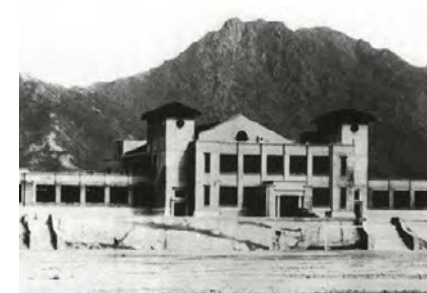
Fig 33: Main Building, Diocesan Boy's School, substantially completed, 1926; subsequently modified (Source: Diocesan Boy's School, 'The House they built from age to age', [links to a pdf], accessed 12 August 2024).
