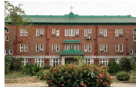
View of the current condition
