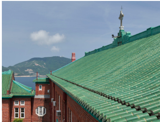
Current condition of existing building
