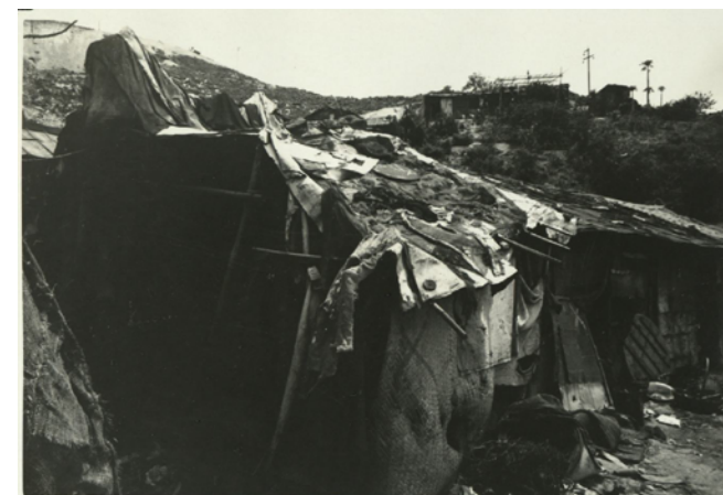
Fig 17: Squatter structures built on the Kwun Tong Refuse dump, April 1955 (Source: Kong Kong Public Records Office, 'Kwun Tong Gallery' [website], Copyright @ 2015 Government Records Service. All Rights Reserved. last revision date: 16 December 2015).
