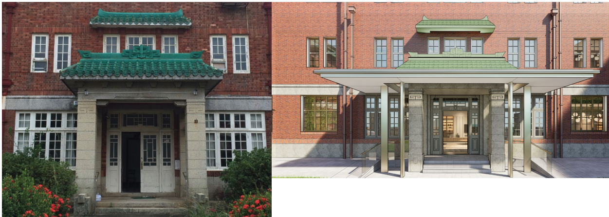
Figure 5.2 New Free-standing Canopy at the Entrance Porch
