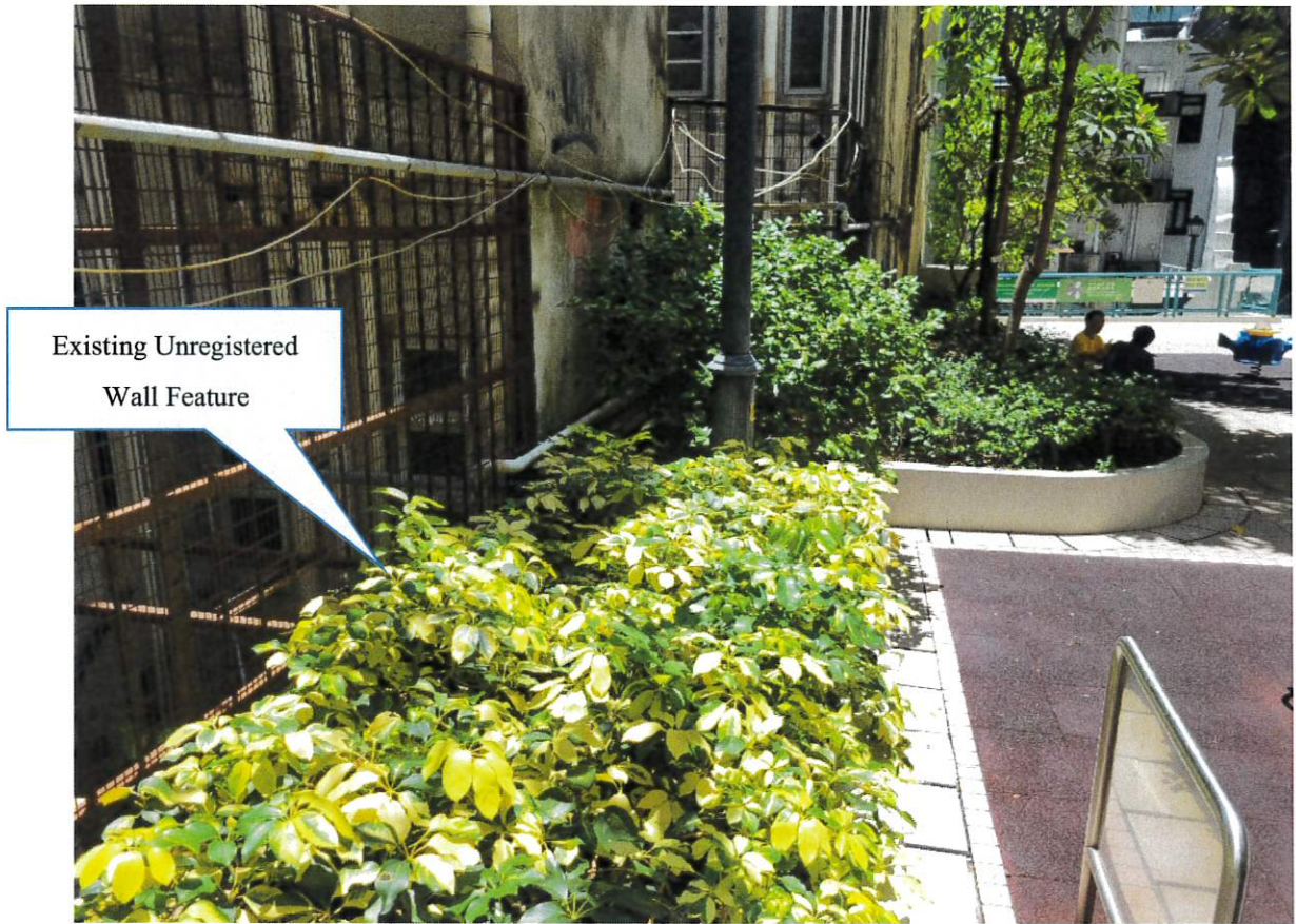
#G08 Crest of an Unregistered Wall Feature at Rear of 156 – 158 Wellington Street
