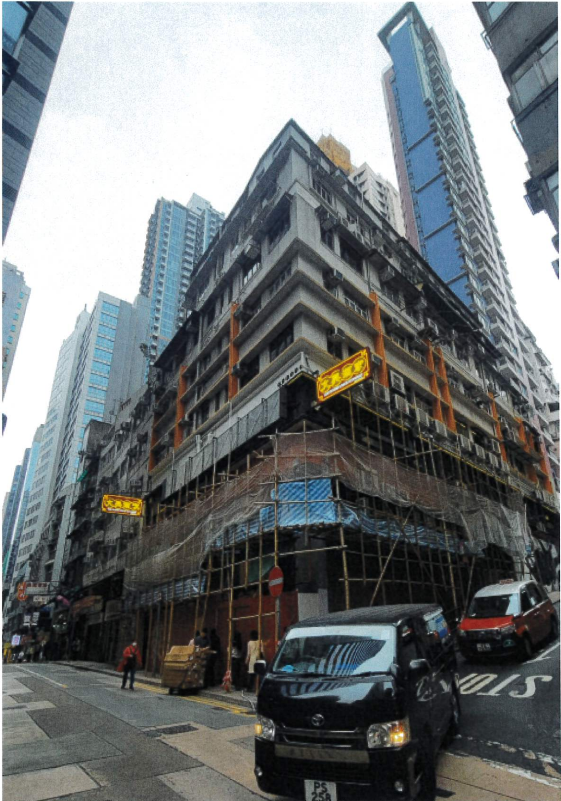
Front View at Wellington Street (152 – 164 Wellington Street)
