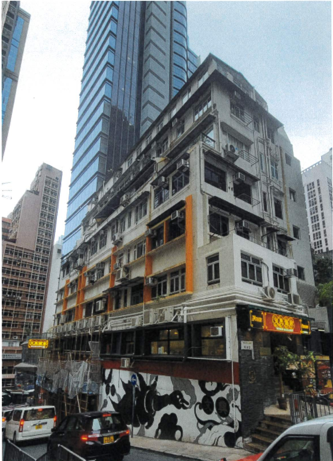
Rear View at Aberdeen Street (160 – 164 Wellington Street)
