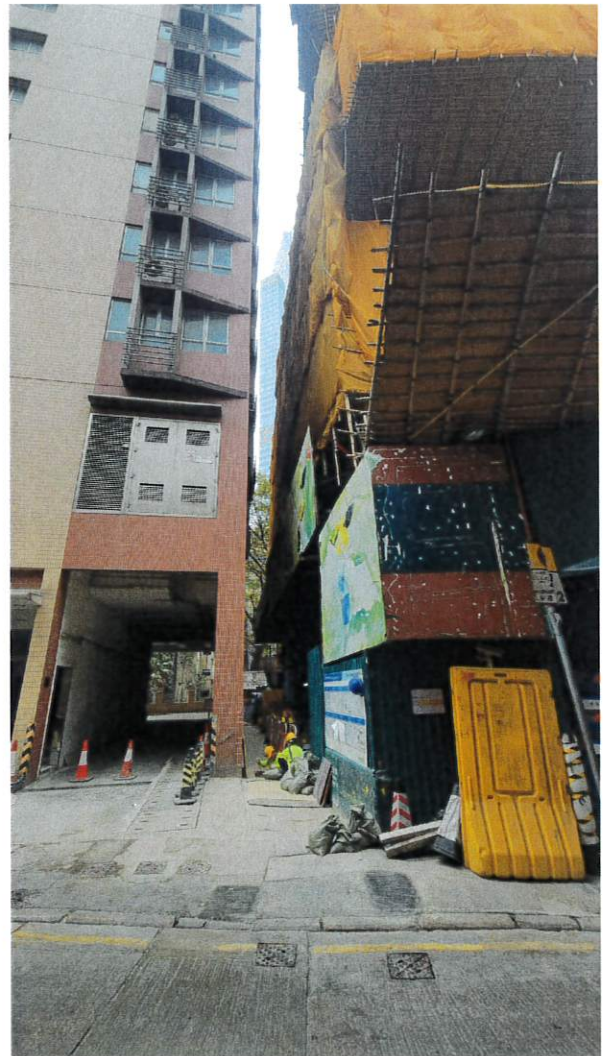
#G07 View at Gage Street (It is suspected that part of the Wall Feature should have been removed or replaced by the New Development at 10 – 14 Staveley Street.)
