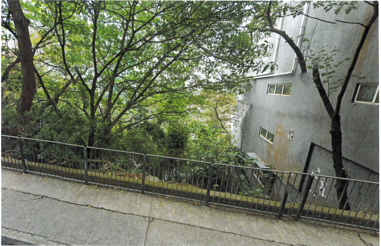
Front View of Area adjoining 60 Tai Hang Road
