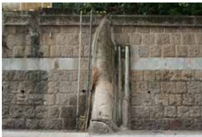
Fig. 3.3.1.11 Existing coping with vermiculated rustication, 2021. (Source: Purcell, 2021)
