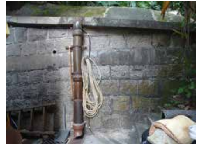
Fig. 4.3.6.2 Glazed clay pipe on masonry wall to the west of Li Hall, St John's Cathedral, possibly from the 1920s during the construction of former Li Hall. (Source: Purcell, 2021)
