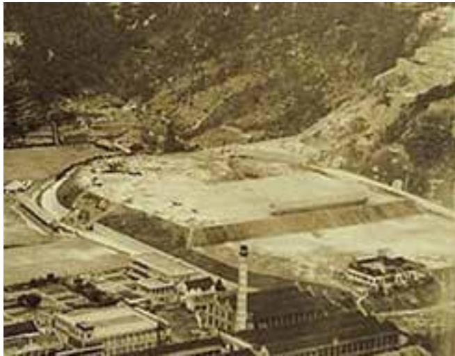
Fig. 3.3.1.15. Aerial photo dated late 1920s or early 1930s showing the largely completed site formation works at Caroline Hill. (Source: H Wong, digitalized by flickr, https://www.flickr.com/photos/35328107@N08/4257151205 )
