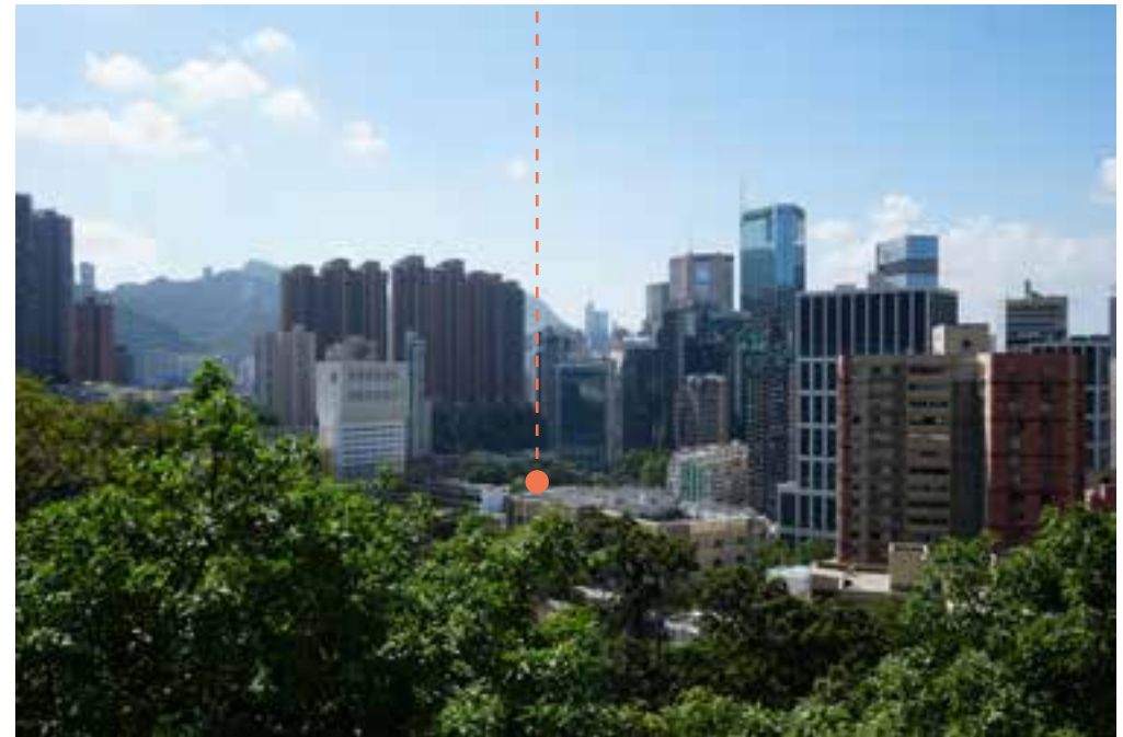
Fig. 2.2.7. Looking west towards the Site from Wang Fung Terrace. Source: Purcell, 2021.
