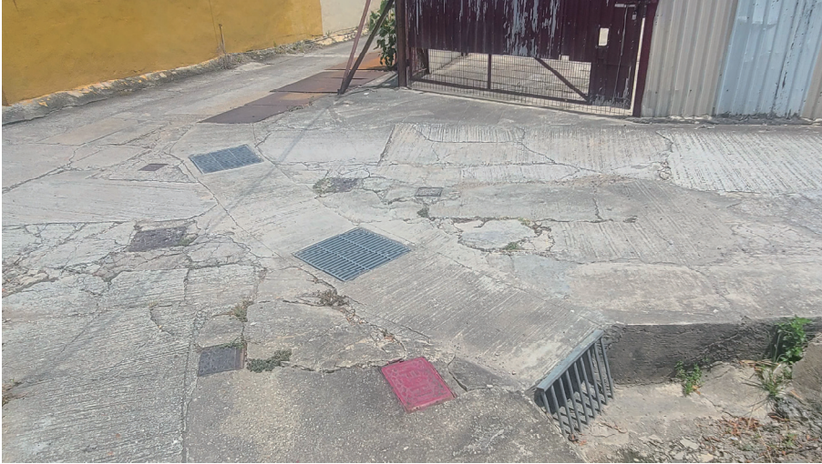
Plate 1 – The inlets of the existing 600UC
