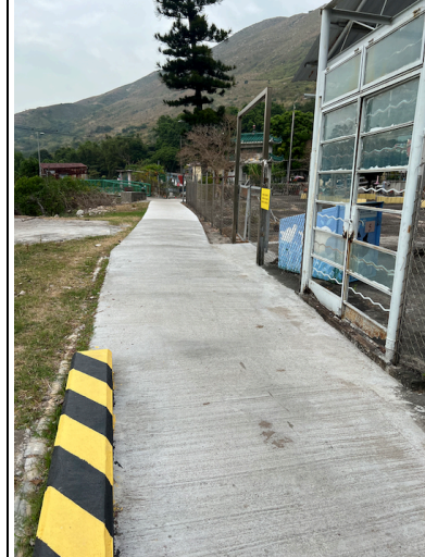
Photo 6 Footpath connecting to entrance of the Monastery
