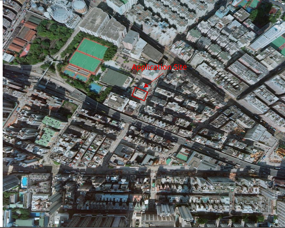
Site Description: Industrial buildings
