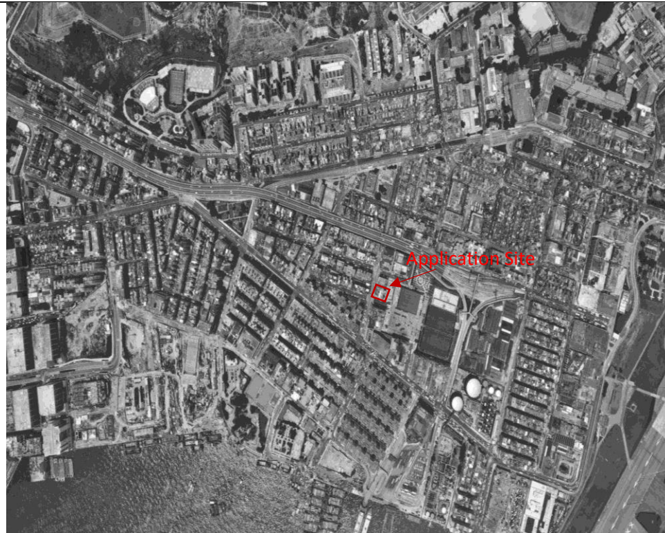
Site Description: Industrial buildings
