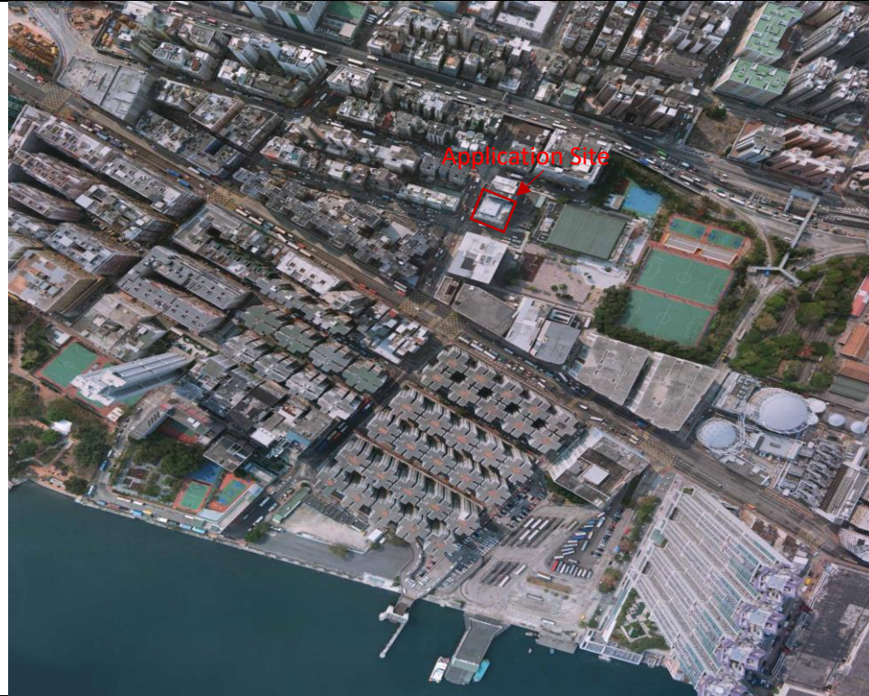
Site Description: Industrial buildings
