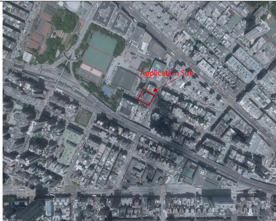
Site Description: Industrial buildings
