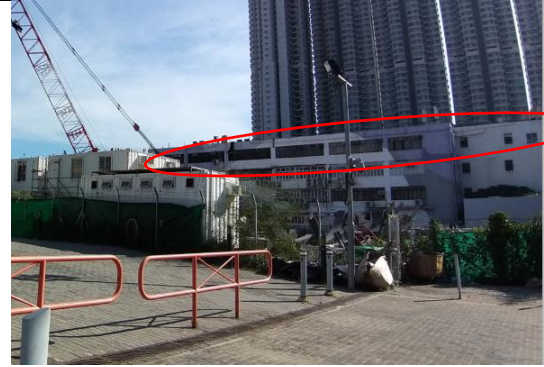
NP_1 to NP_18: Cooling Tower/Air Cooled Chillers at Newport Centre Phase 1 & 2 (To be redeveloped by URA)
