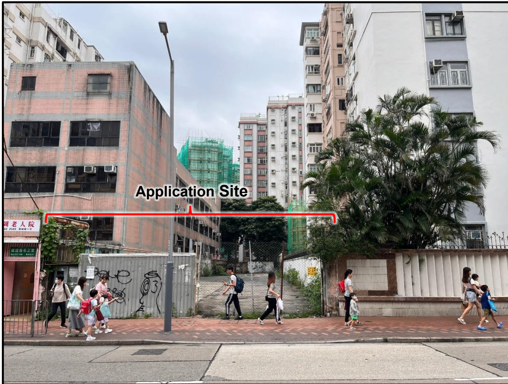
Figure 2.2a Site Photo (Viewing from Prince Edward Road West)
