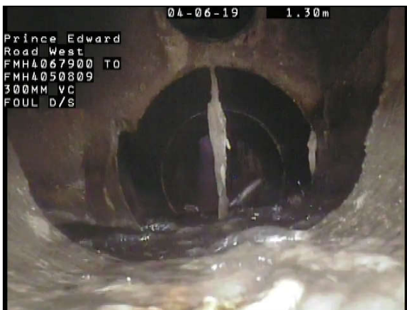
Photo Ref. : 021 Video Tape : 0001, 0:00:37 Observation : General Photograph
