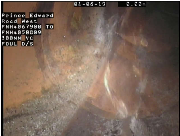
Photo Ref. : 019 Video Tape : 0001, 0:00:32 Observation : General Photograph
