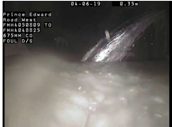
Photo Ref. : 024 Video Tape : 0001, 0:00:59 Observation : General Photograph
