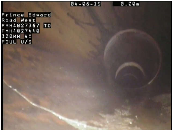
Photo Ref. : 039 Video Tape : 0001, 0:00:43 Observation : General Photograph
