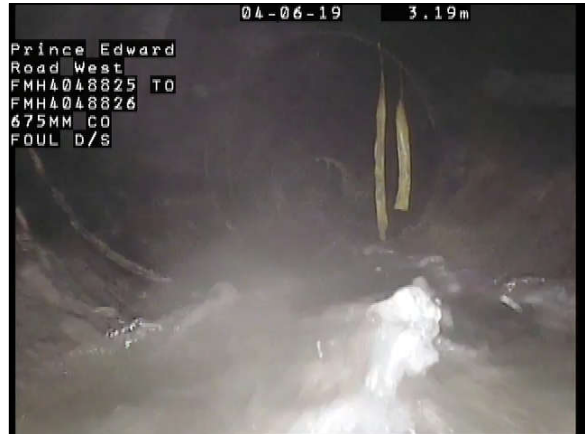
Photo Ref. : 027 Video Tape : 0001, 0:03:19 Observation : Fracture Circumferential, from 06 to 09 o'clock
