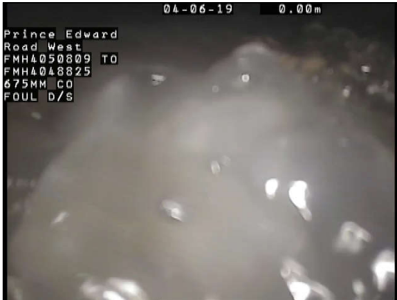
Photo Ref. : 023 Video Tape : 0001, 0:00:55 Observation : General Photograph
