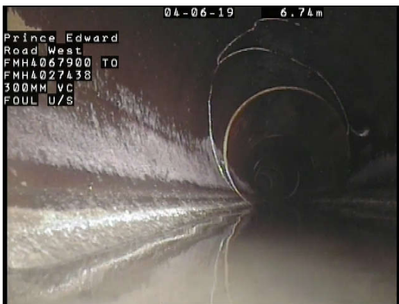
Photo Ref. : 014 Video Tape : 0001, 0:01:33 Observation : Fracture Circumferential, from 07 to 04 o'clock
