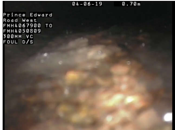
Photo Ref. : 020 Video Tape : 0001, 0:00:36 Observation : General Photograph
