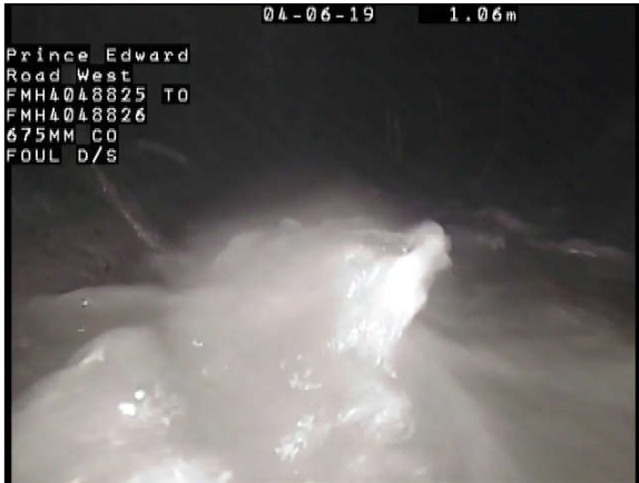
Photo Ref. : 026 Video Tape : 0001, 000054 Observation : General Photograph
