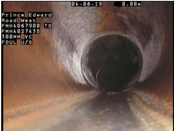
Photo Ref. : 008 Video Tape : 0001, 0:00:37 Observation : General Photograph
