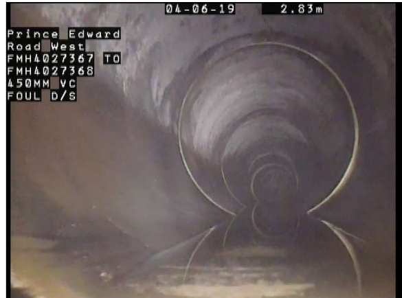
Photo Ref. : 036 Video Tape : 0001, 0:01:17 Observation : General Photograph
