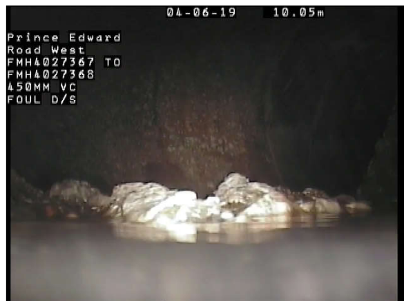
Photo Ref. : 038 Video Tape : 0001, 0:01:52 Observation : General Photograph
