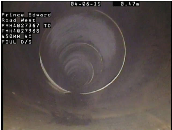
Photo Ref. : 035 Video Tape : 0001, 0:01:03 Observation : General Photograph
