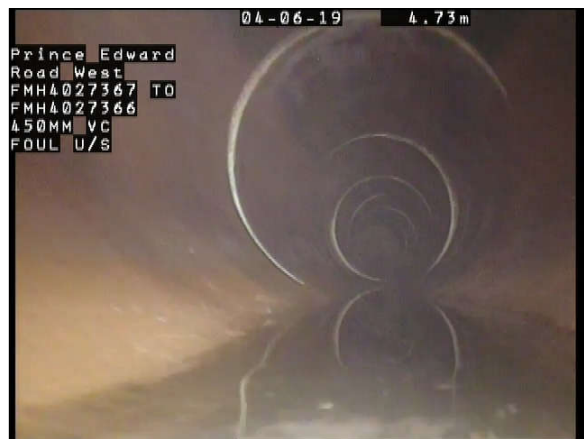
Photo Ref. : 048 Video Tape : 0001, 0:01:06 Observation : General Photograph
