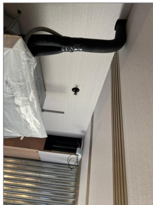
Photos 2.2 & 2.3: The Automatic Sprinkler System within the Premises
