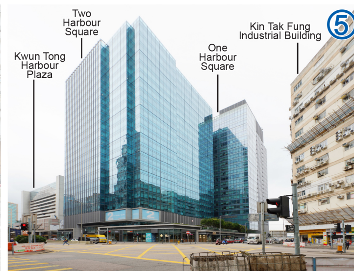
High-Rise Commercial Building viewed from the corner of Tsun Yip Street and Wai Yip Street
