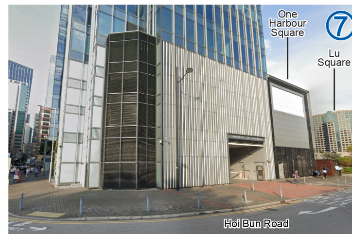
Car Park Entrance of One Harbour Square at Hoi Bun Road
