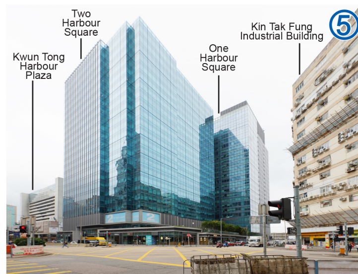
High-Rise Commercial Building viewed from the corner of Tsun Yip Street and Wai Yip Street
