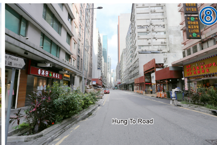
Industrial Clusters viewed from the South-east of Hung To Road
