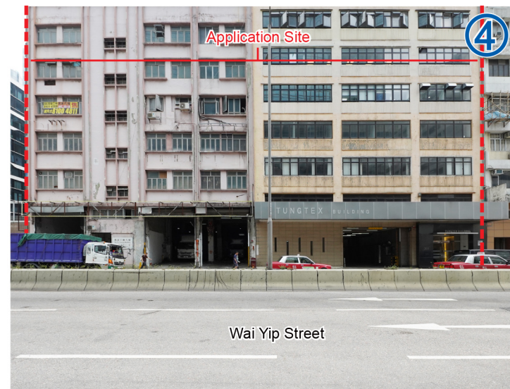
Existing Condition of the Application Site viewed from Wai Yip Street
