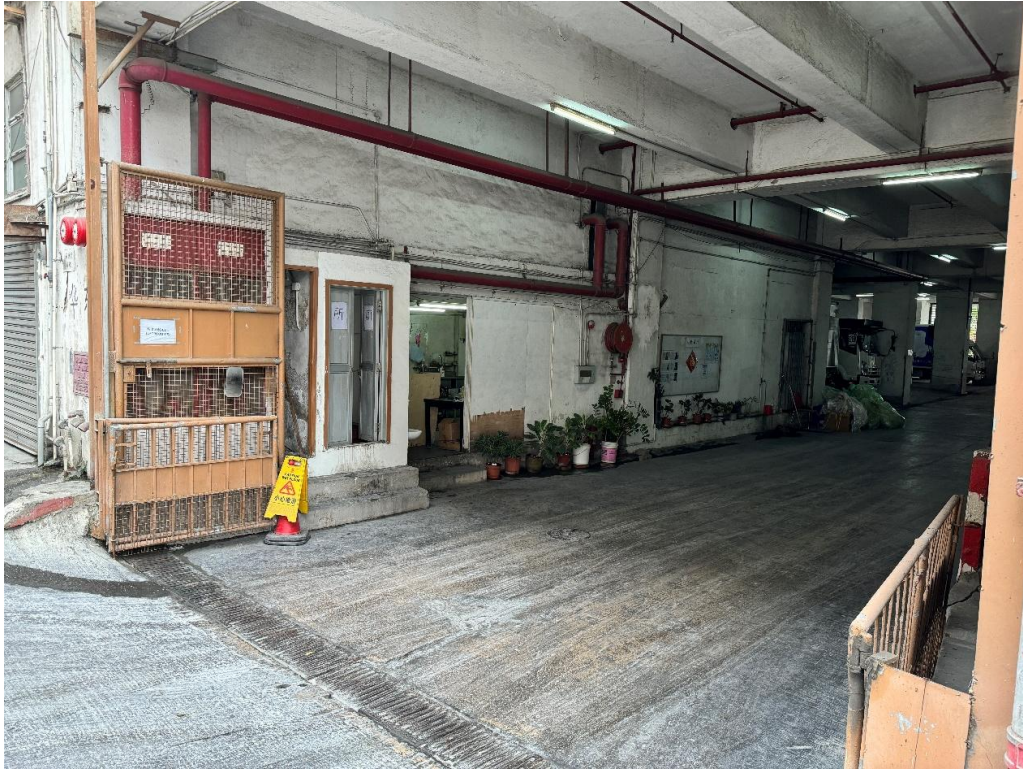
Building entre area, paved with good condition
