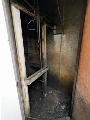
Photo 45 Storeroom at LG/2
