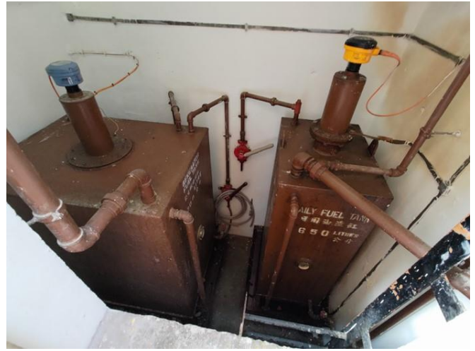
Photo 32 Oil Tank Room at LG/1
