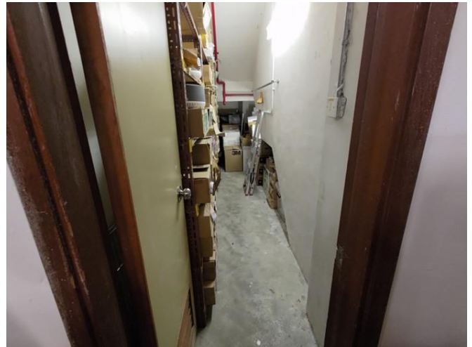
Photo 16 Storeroom at G/F
