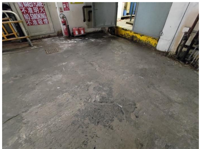
Photo 48 Boiler Room Fire Escape Corridor at LG/2
