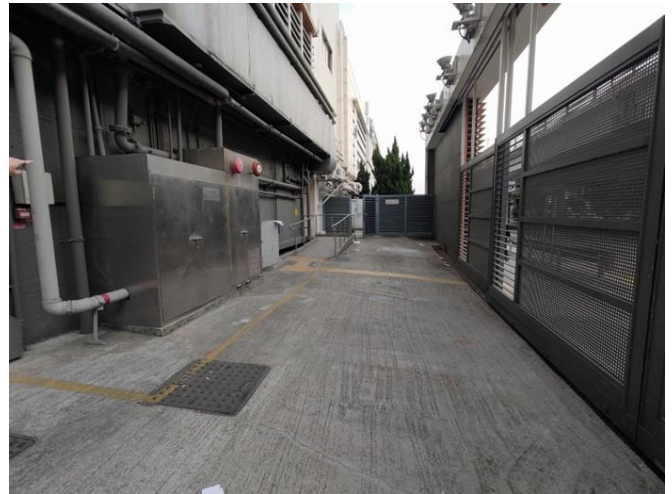
Photo 58 Loading and Unloading Bay at LG/2
