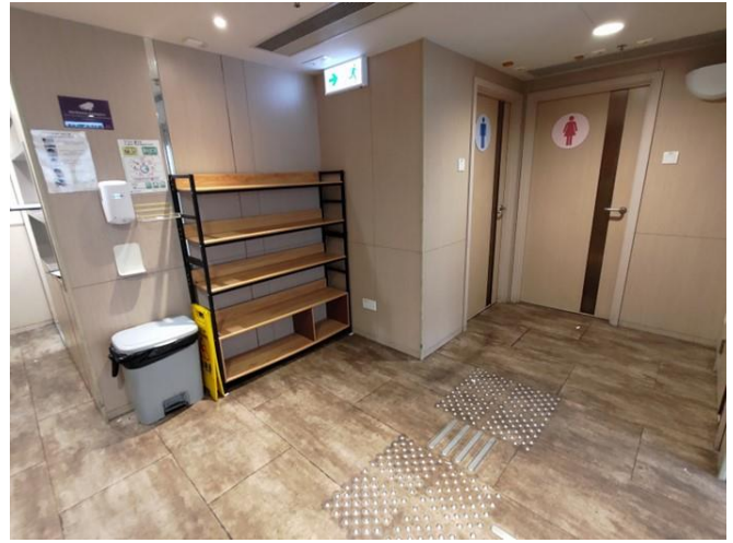
Photo 26 Canteen Entrance at LG/1
