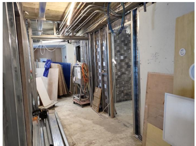
Photo 30 Renovation Works Area at LG/1
