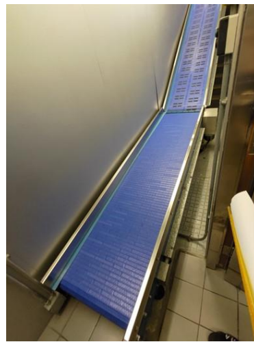
Photo 40 Equipment Room at LG/1
