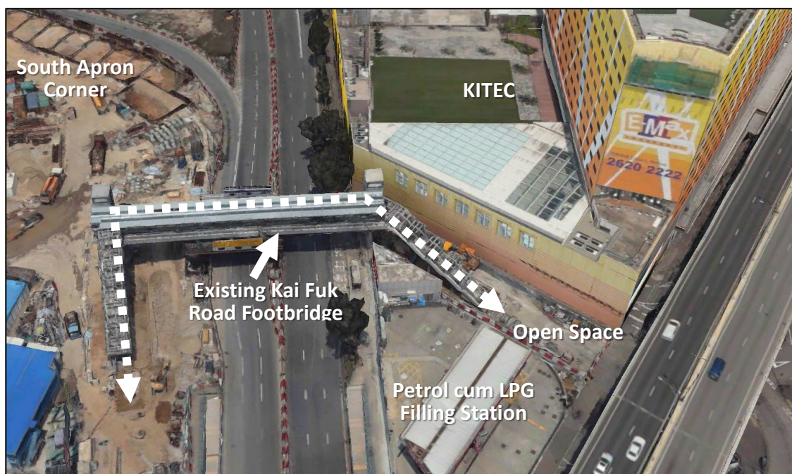
Figure 2.7: Existing government footbridge across Kai Fuk Road
