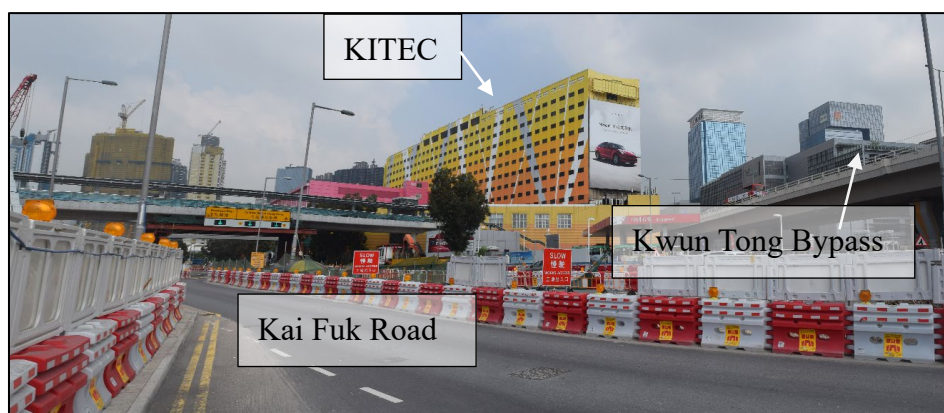
Photo 3.2 Site Photo (facing the eastern side of the Site)
