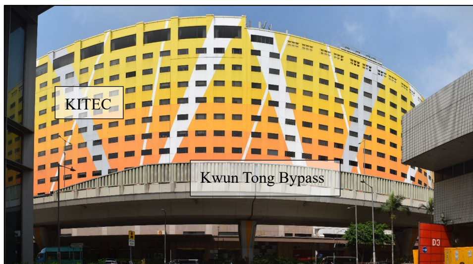
Photo 3.1 Site Photo (facing the eastern side of the Site)
