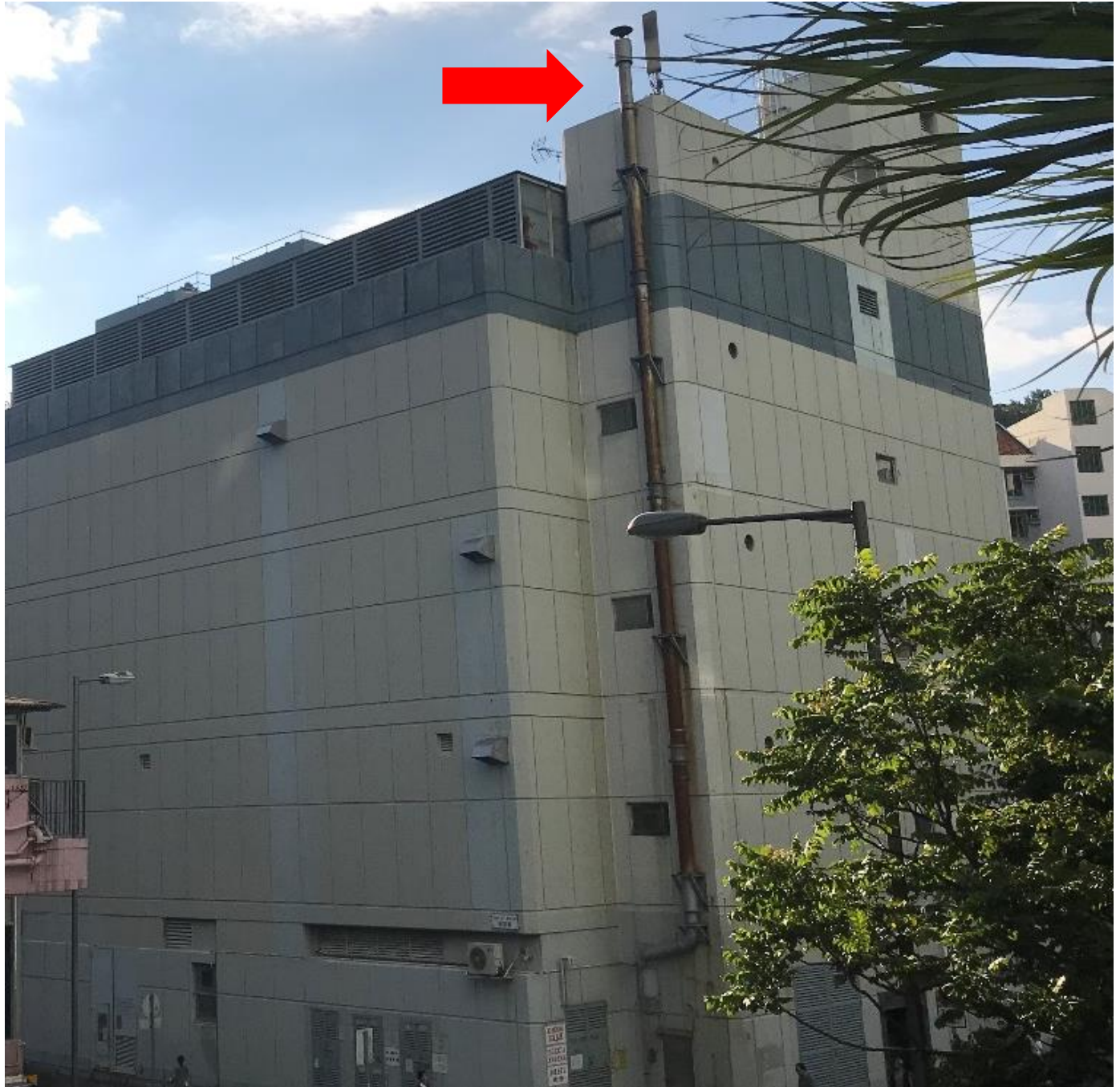
PCCW Telephone Exchange Building
