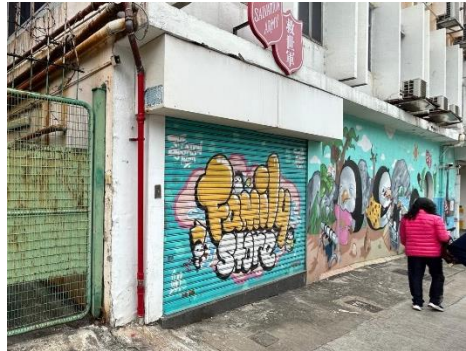
Front view of the Subject Premise
