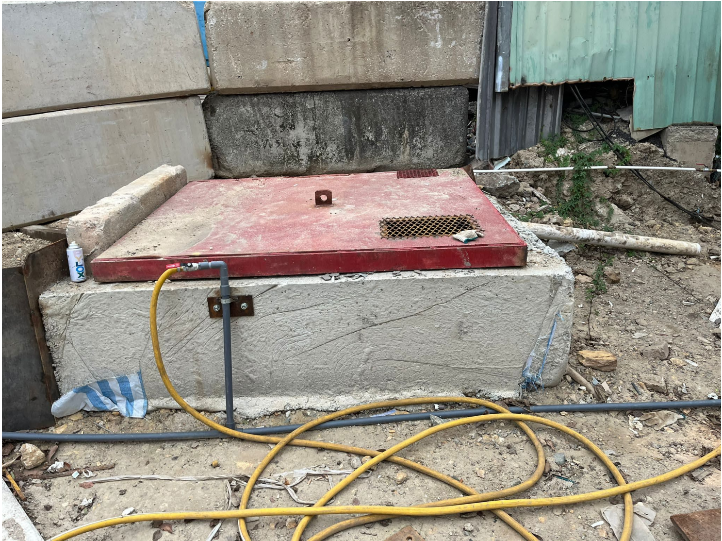
Figure 2. Existing Catchpit with Sand trap #1
