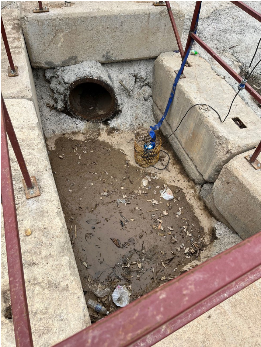
Figure 3. Existing Catchpit with Sand trap #2
