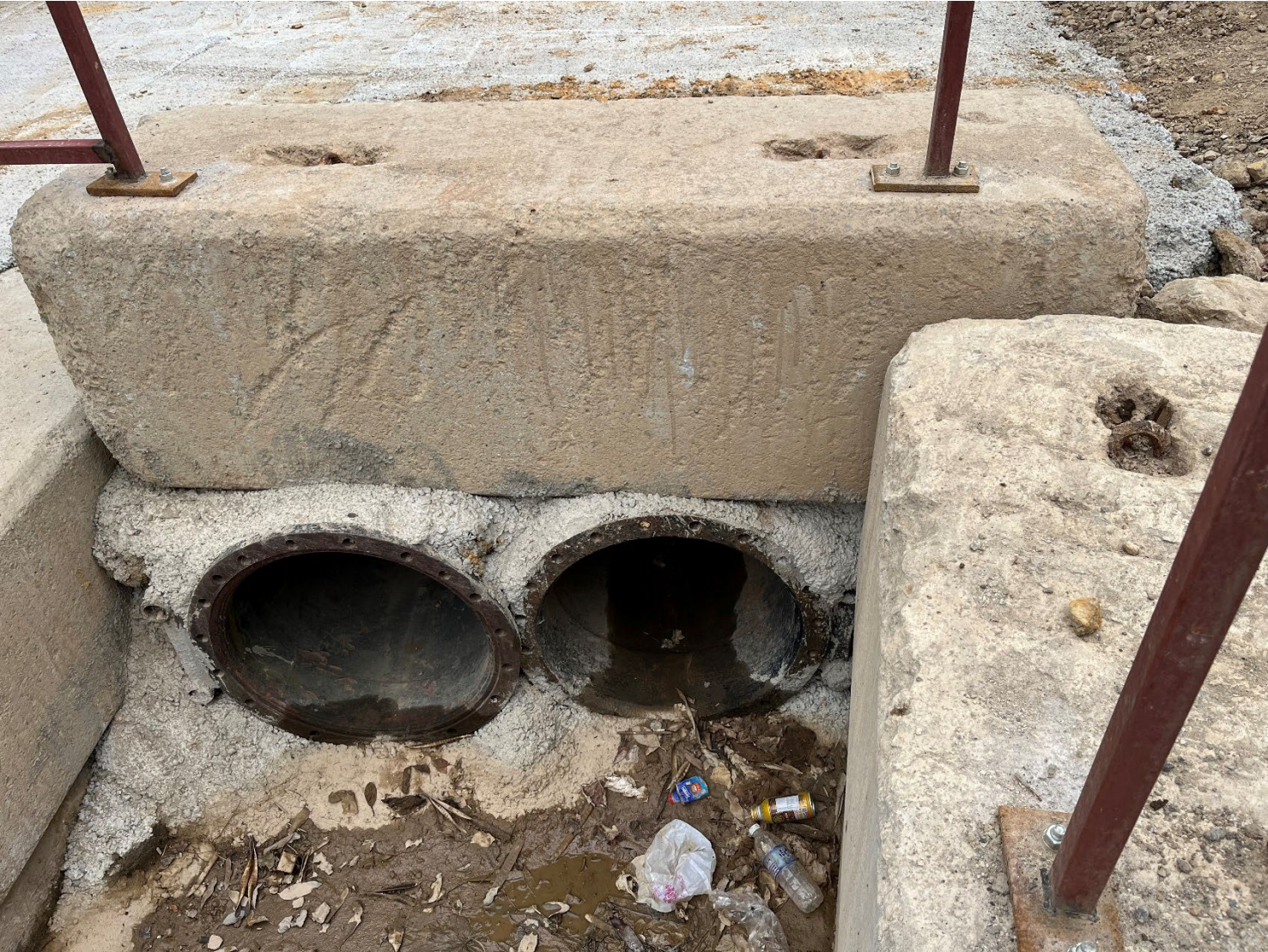
Figure 4. Existing Catchpit with Sand Trap #2
