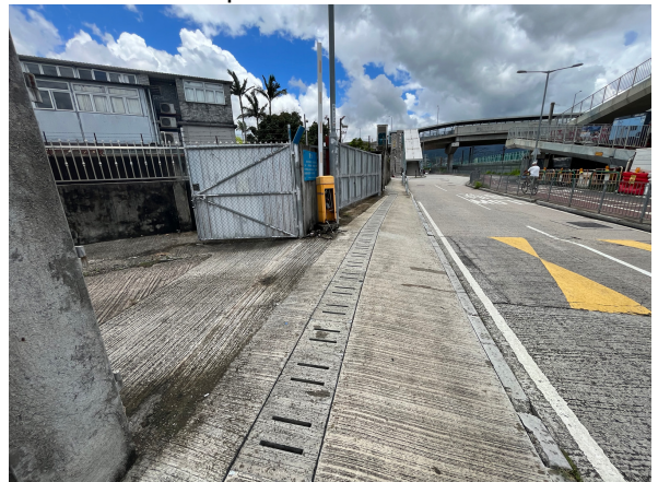
Photo 6: Accessible via local track.
