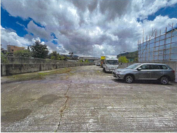
Photo 3: South-western part of the site.
