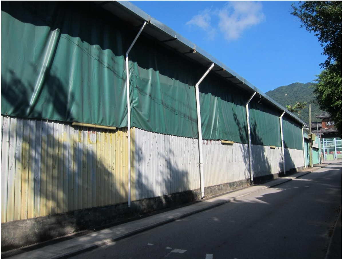
Photo 1: Existing gutters at the roof of the warehouse
