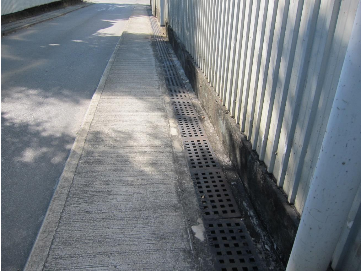
Photo 4: Existing u-channel on the ground
