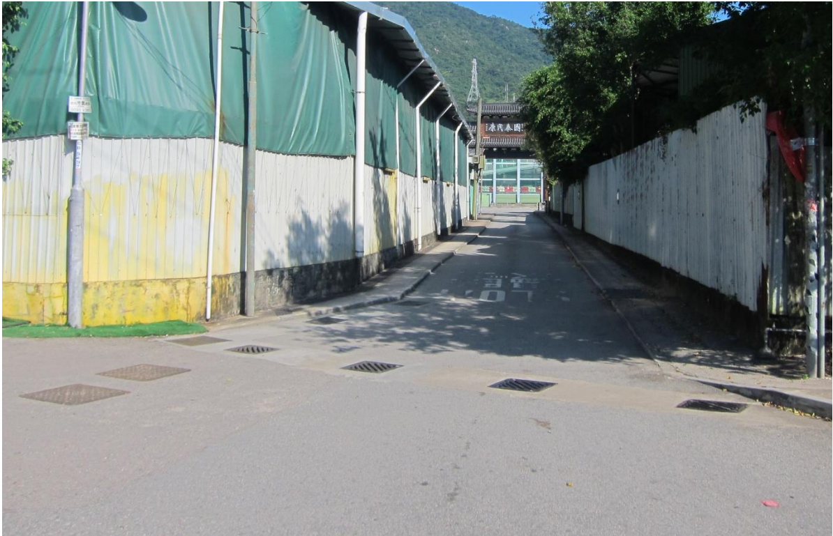
Photo 6: Discharge to existing Government pipe
