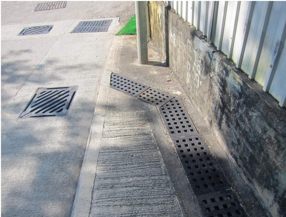
Photo 5: Existing u-channel on the ground
