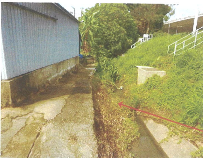
Photo No. A6
