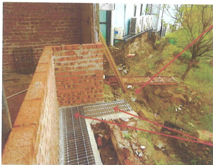
Photo No. A6
