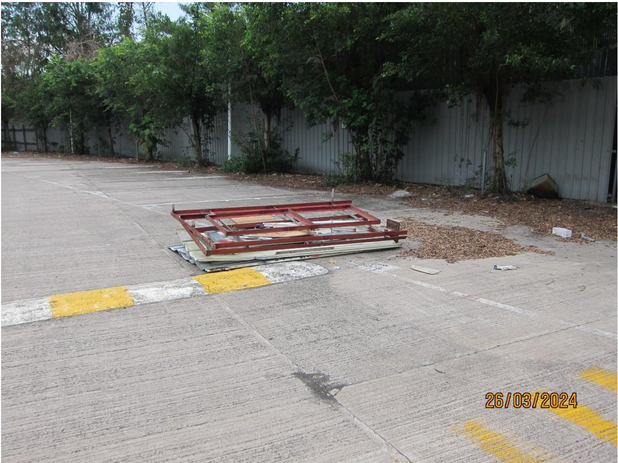
Photo 2 The meter room erected on Lot 1494 in DD76 has been demolished
